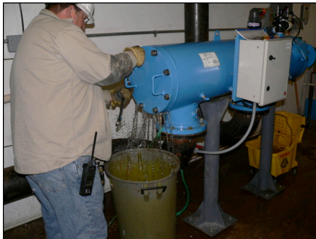
• Figure 7: Opening the filter housing to change the filter cartridge
