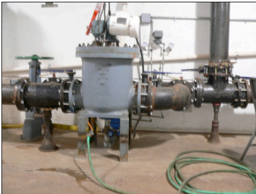
• Figure 3: Existing Hayward strainer upstream of BallastSafe Filter
