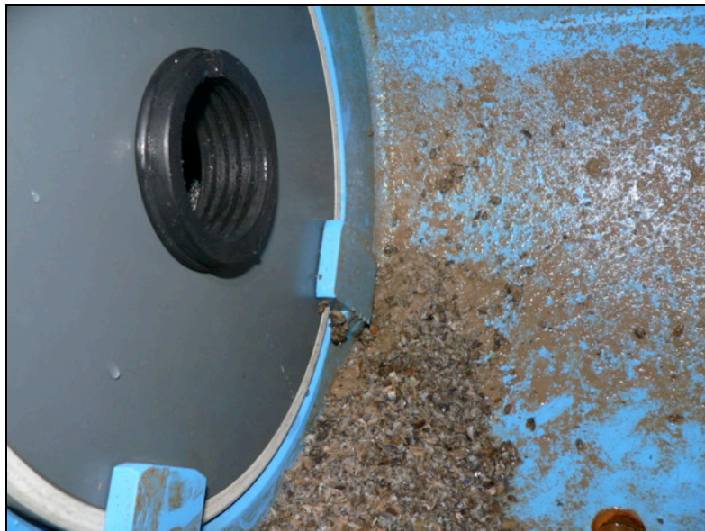
• Figure 11: Inside of backwash chamber showing typical debris removed from water stream
