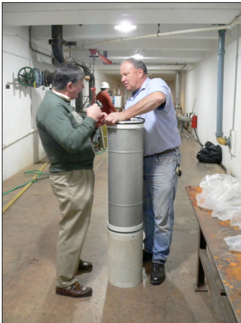
• Figure 6: Filter cartridge being prepared for change-out
