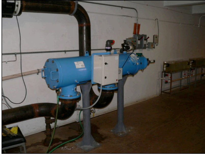
• Figure 4: Ballast Safe Filter installed at Parker
